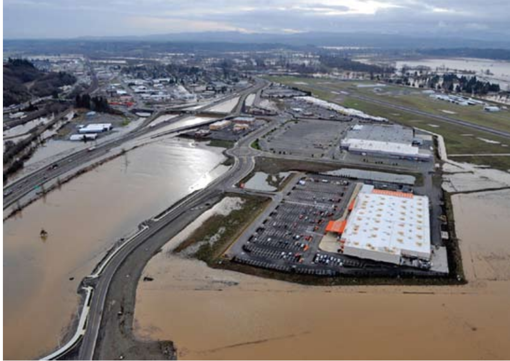
Flood waters turn Chehalis Wal-Mart and Home Depot parking lots into islands. I-5 is in the upper left.
