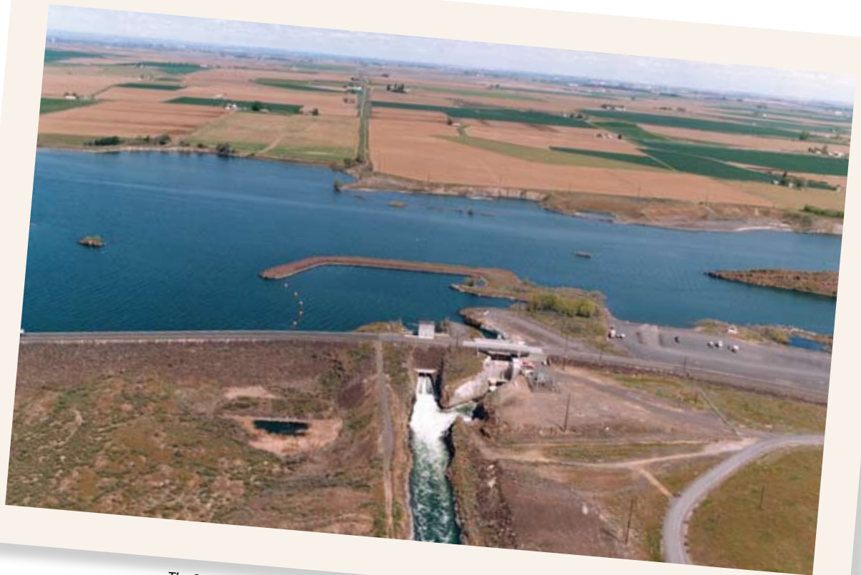
The Potholes East Canal Headworks Project, operated by Grant PUD since 1990, generates 6.5 megawatts of power using water flow in the irrigation canal.
