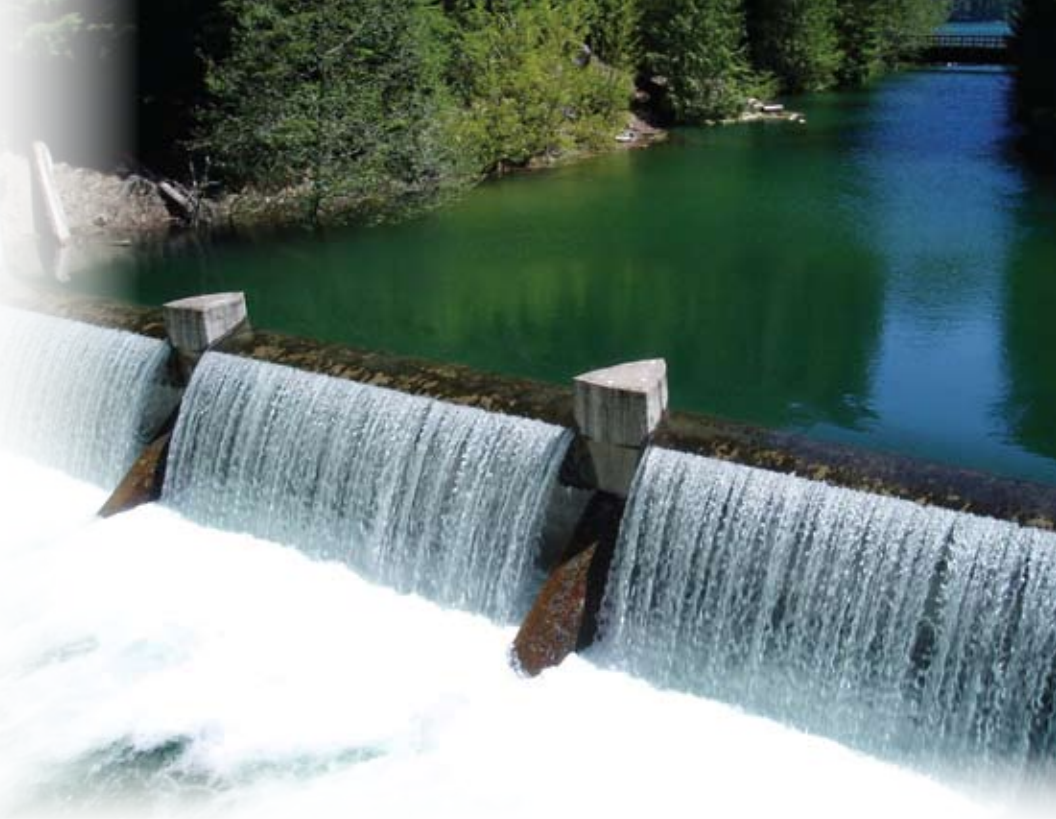
Diversion dam on Lake Creek channels water from Packwood Lake to powerhouse 1,800 feet below the lake.
